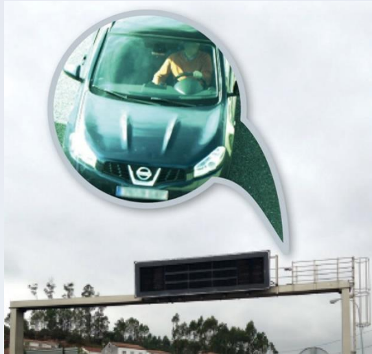
Illustration 102. Artificial vision cameras to control the use of the belt. Source: DGT Magazine
