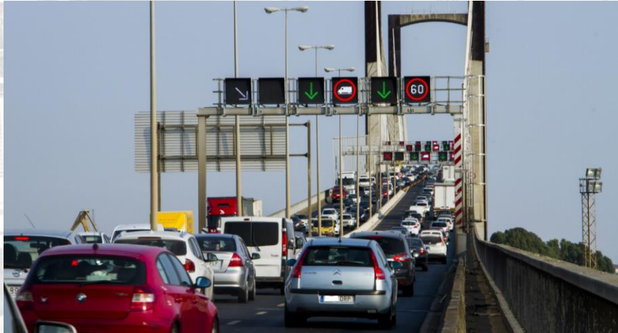
Illustration 25. Reversible lane V Centenario Bridge. Source: DGT
