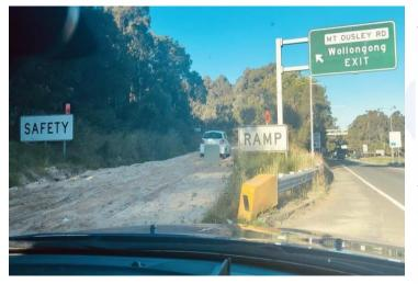
Truck 'arrester beds' or 'sand traps' are designed to stop heavy vehicles at the bottom of steep hills if they run out of brakes.
